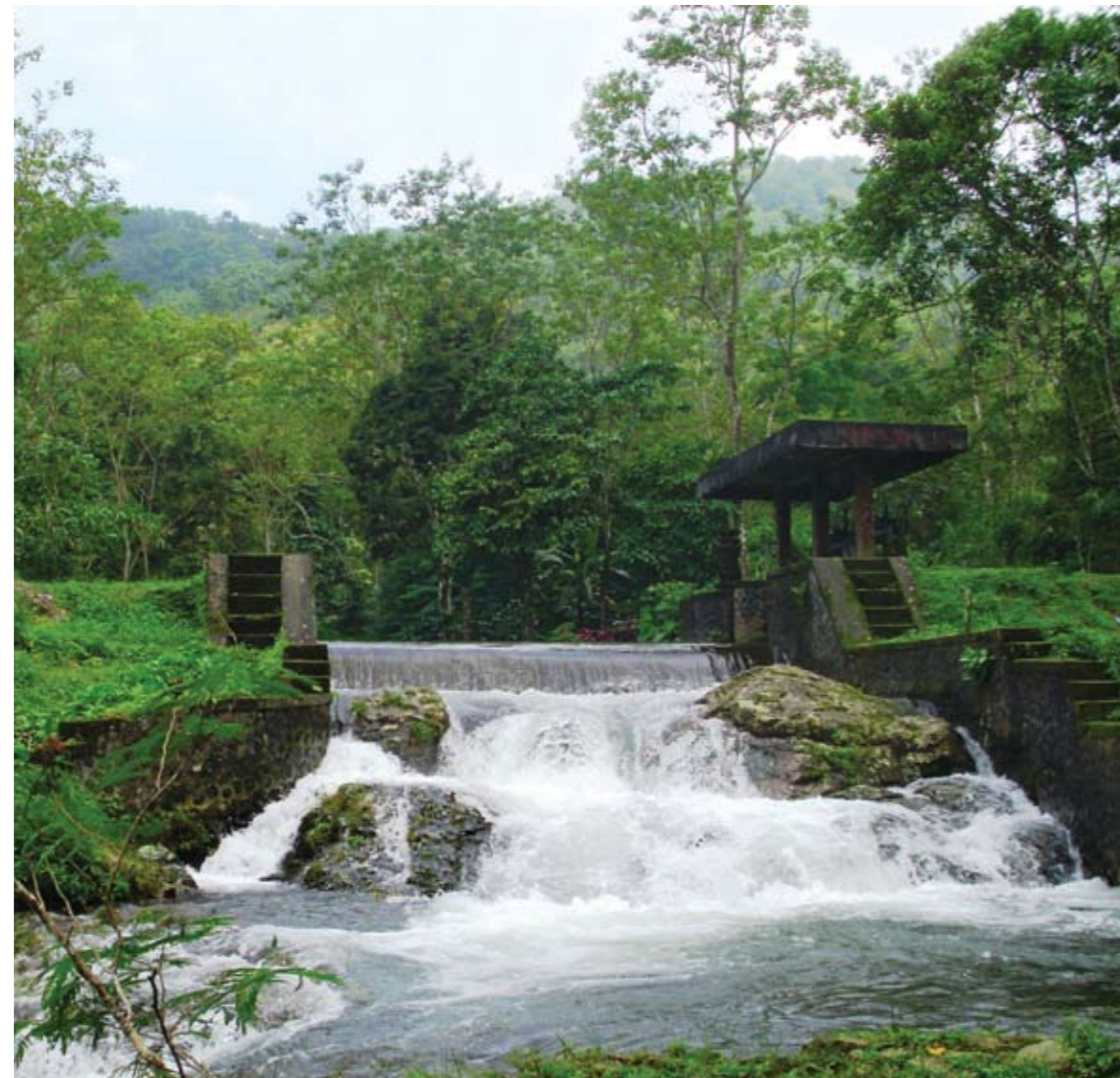
Micro hydro (5m 3 /sec) of public work in Buleleng, Bali
